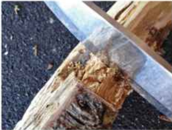
Make a \frac{1}{8} "– \frac{1}{4} " cut down either side of the notch with your blade, then pop that small section out.
